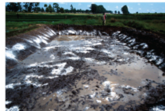
Lime pond bottom and all dykes
