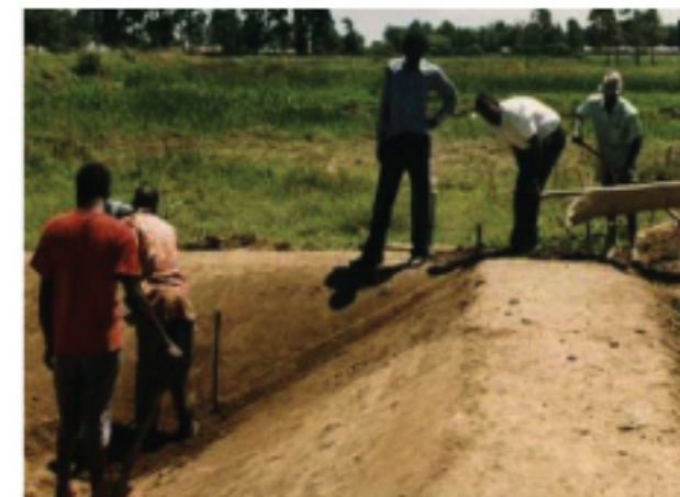
Pond construction with well constructed dyke slopes
