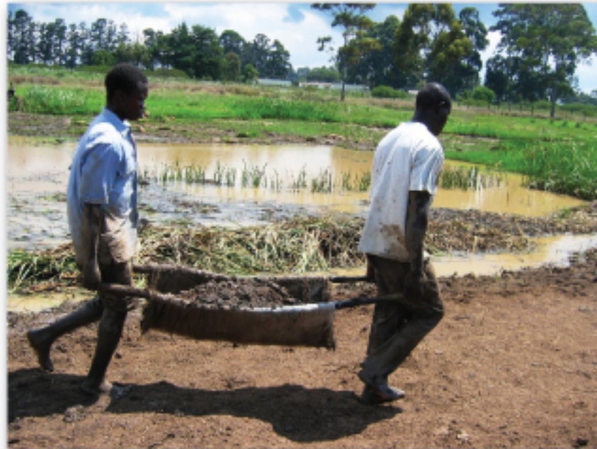
Compacting core trench reduces water loss through dykes
