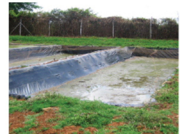
Using liners in poor soils
