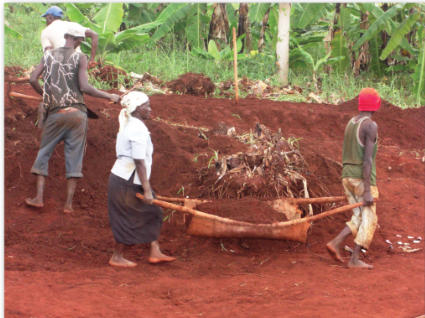
Transporting soils to the dikes or away from the pond dykes
